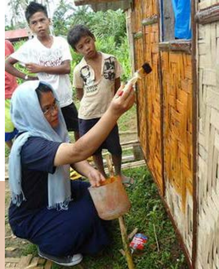
Philippines Rebuilding shelters after typhoon destruction
